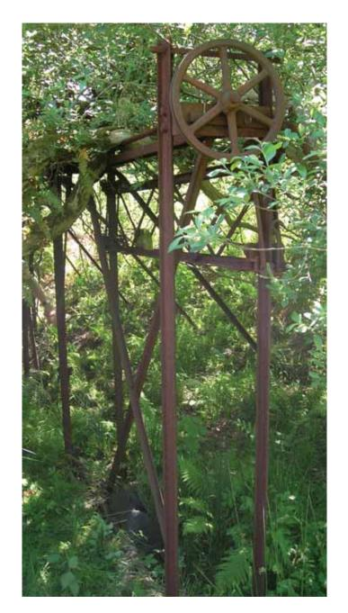
One of six target frames on a 600-yard rifle range surviving in thick undergrowth near Dolgellau, Gwynedd. Built in World War I and also used during World War 2, each castiron target frame enabled a target to be raised, fired at, lowered and repaired or replaced (© Medwyn Parry).
