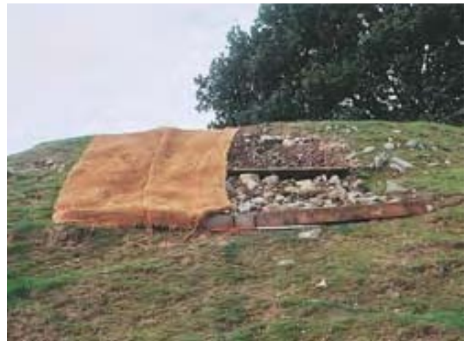
The erosion scars (above left) on Aber Motte in Gwynedd have now been repaired under a Tir Gofal capital works programme (above). The repairs will ensure that the shape of the motte is restored and the grass is allowed to recover (opposite).
